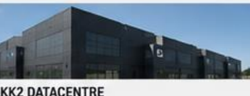
LKK2 DATACENTRE Digital Reality 📍 Lagos State
