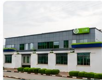
DEVELOPMENT BANK OF NIGERIA, ABUJA
