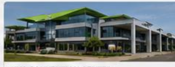
UYO CONVENTION CENTER Craneburg Construction 📍 Akwa Ibom State
