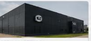
LG03 DATACENTRE VACC TECHNICAL 📍 Lagos State
