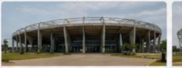
GMK STADIUM PROJECT ITB - Hitech Benin 📍 Kaduna State
