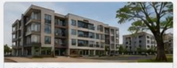
B39 PROJECT El-alan Construction 📍 Lagos State
